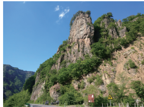
图 3 四道沟镇 08 号潜在崩塌灾害 Fig.3 No.8 potential collapse hazard in Sidaogou Town
